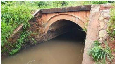
Photos 53: Pont Arche
